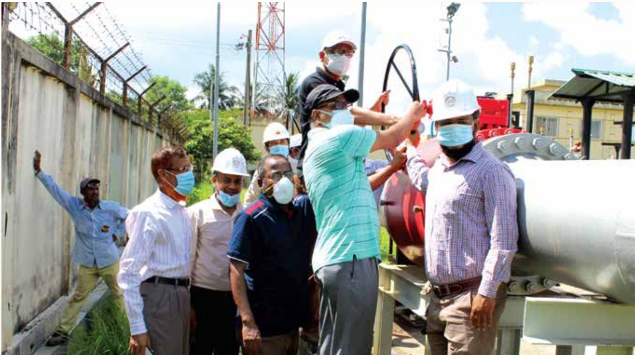
Gas Commissioning to NBBL's temporary RMS
