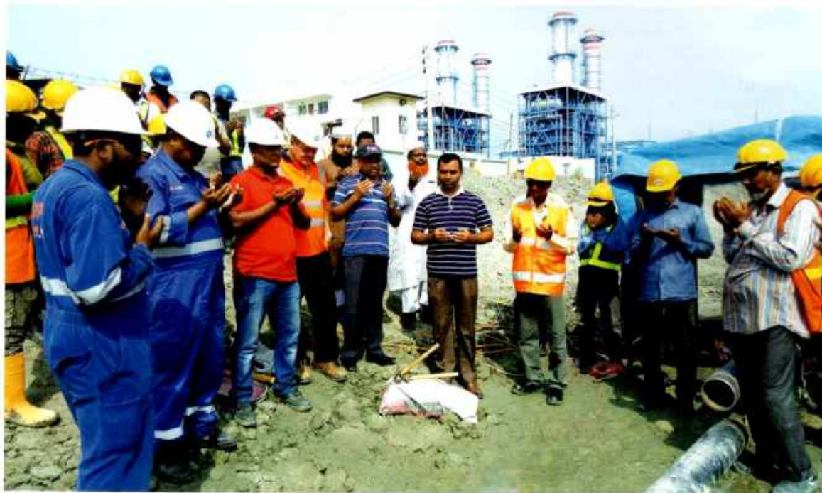
Inauguration of Pipeline Construction for 95 MW Rental Power Plant at Borhanuddin
