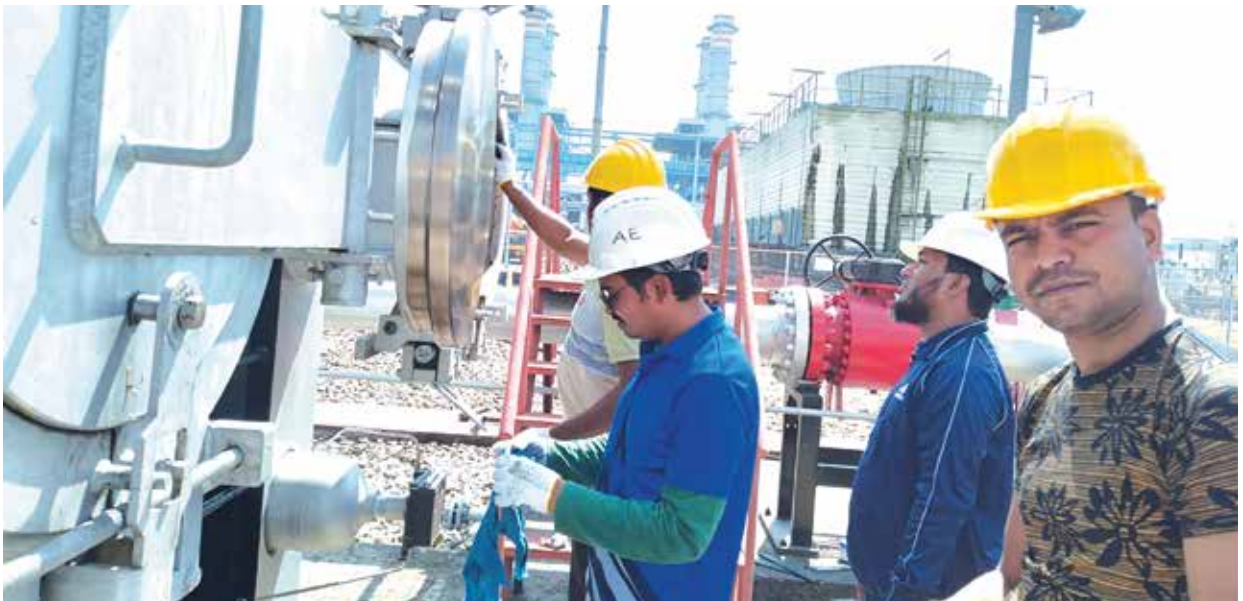
Regular Maintenance of 225 MW RMS, Bhola
