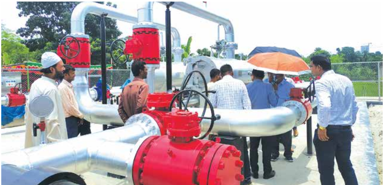
Construction of DRS, Kushtia
