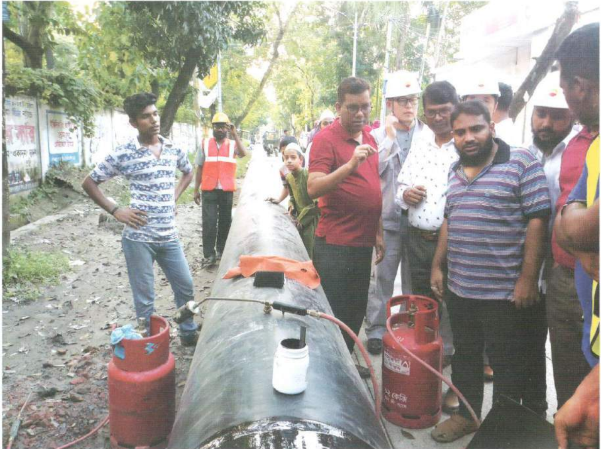
Construction of Line pipe for Gas Connection to 225 & 800 MW Power Plant
