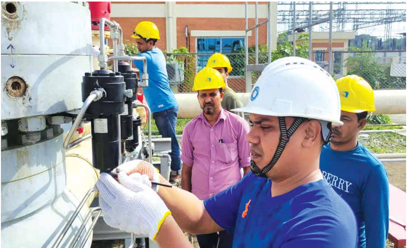
Bheramara RMS Maintenance activities
